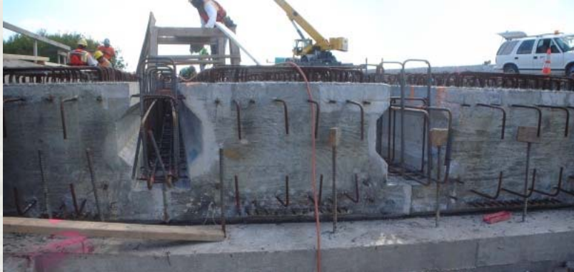
Fish Creek Precast Plank Beam Ends
