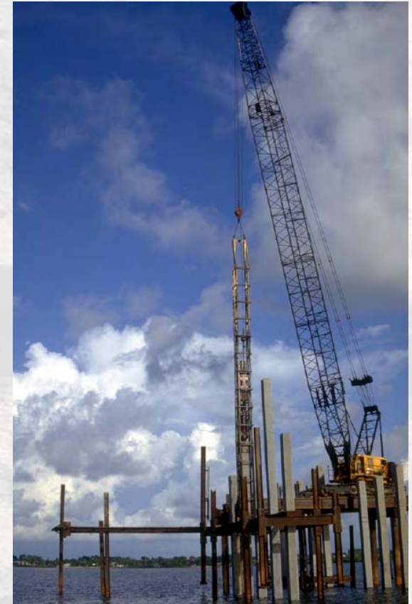
Bayside Bridge Top-Down Construction
